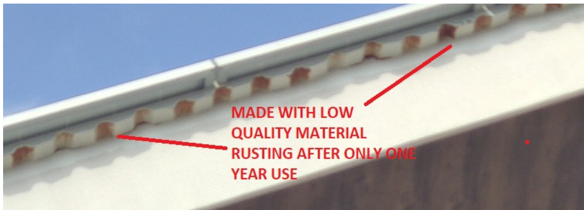
ROOF RUSTING AND IS ONLY ONE YEAR OLD
