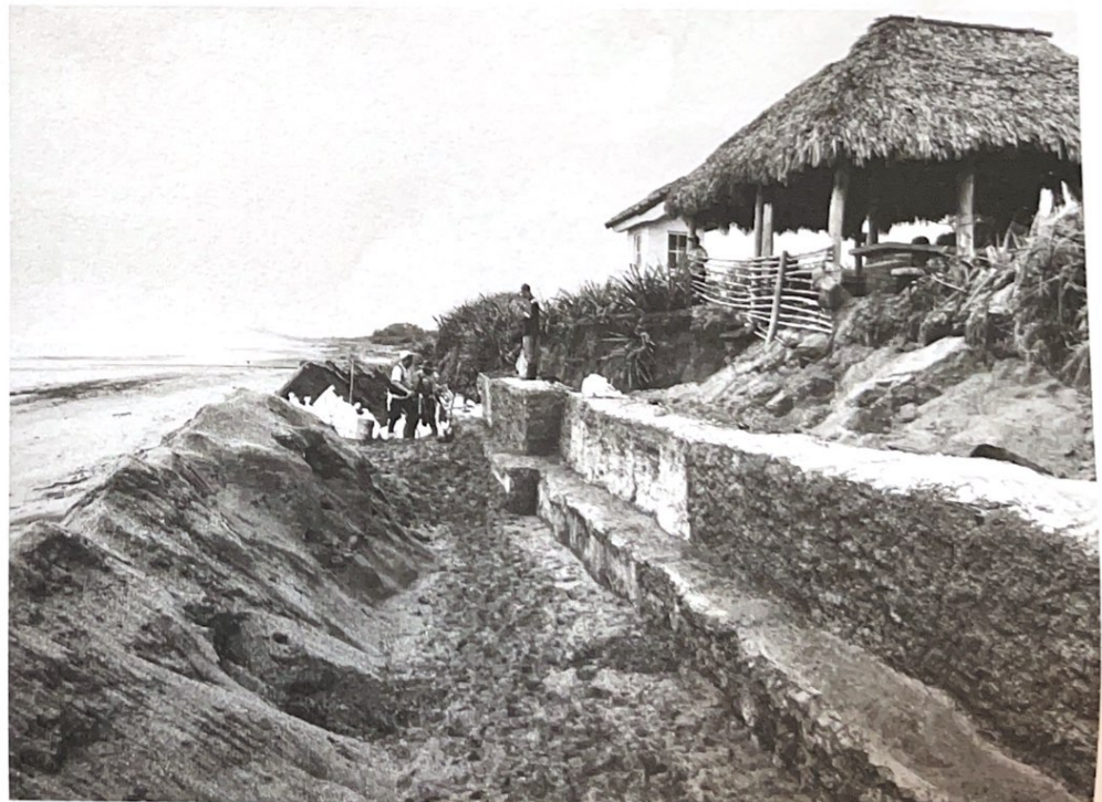
Workers building a protective wall on the north beach by Asuchillo.
